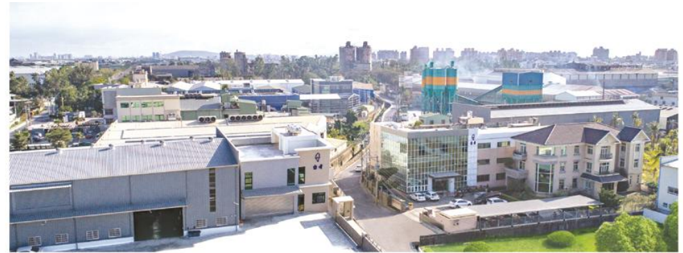
▲台湾厂全景 FACTORY VIEW OF TAIWAN
